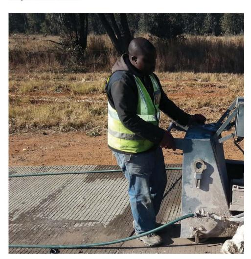
Removal of the old silicon joints which are no longer waterlight.
