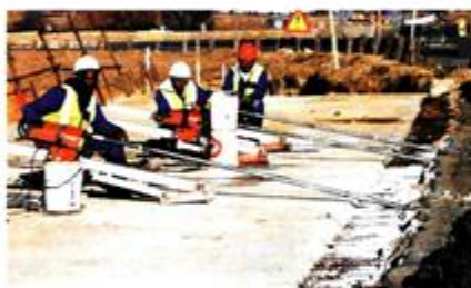
Three drilling machines running 2,4-m-long, 41-mm barrels.
