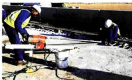
Accurate collaring of the 41-mm bit was crucial.
