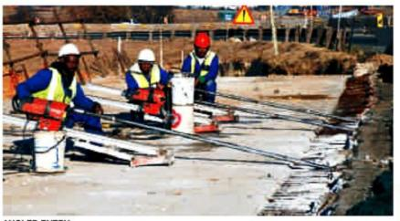
A total of 560 holes were drilled to allow the three bridges to be linked by reinforced steel bars
