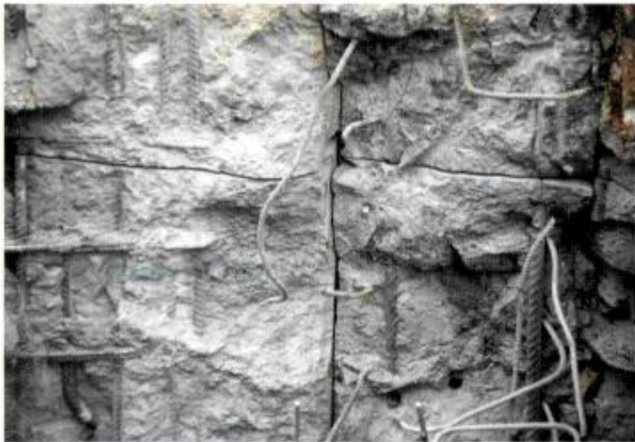
Perfect cuts made using Razor wire verses the rough surface left from conventional breaking.
