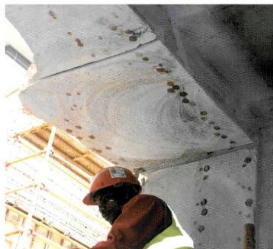
1m thick cut showing Y32 steel cut by the Razor wire.
