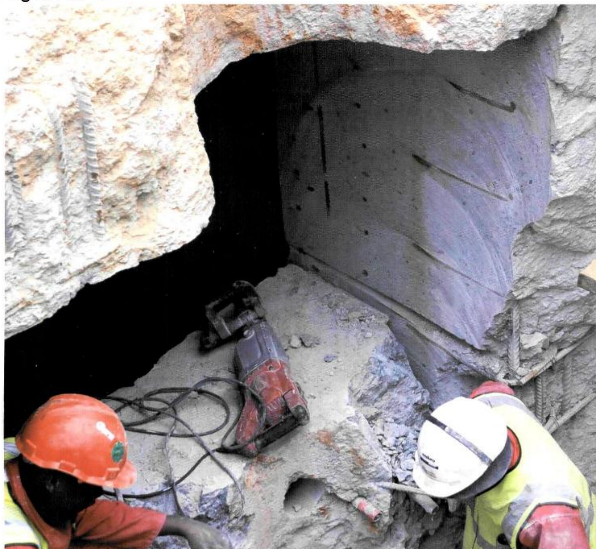
Accurate cut through heavily reinforced concrete.
