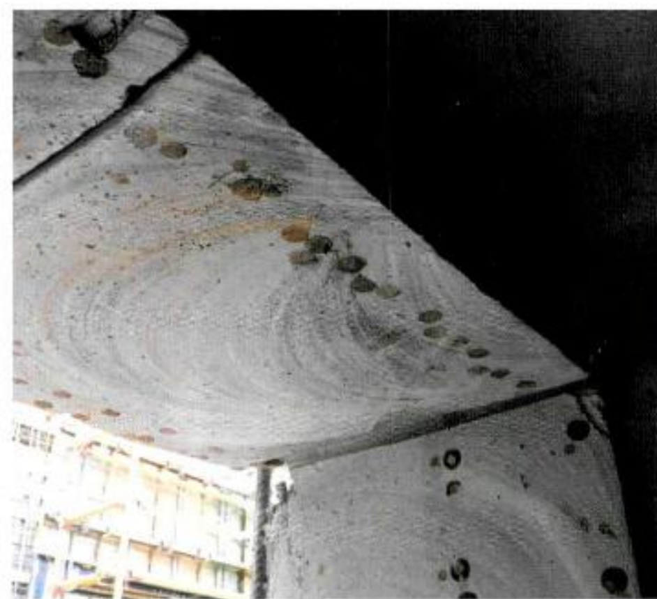
Heavily reinforced concrete showing Y32 steel.
