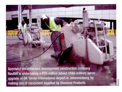
LaserPro CC38 segmented blades. The CC38 blade is designed for specialised contractors for full depth slab cutting of very hard concrete, and has proven to be ideally-suited to Raubex Construction in the application of this project."
