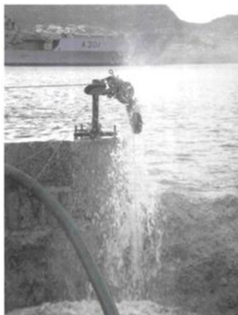
A 360-degree swivelling head allows for horizontal and vertical cutting with the wire.
