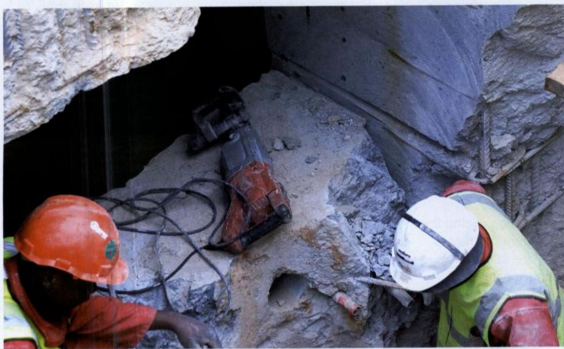
Diamond Products' Razor reinforced diamond wire cuts through reinforced concrete accurately and without causing vibrations in the structure.
